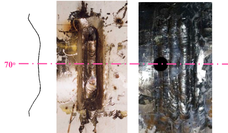
Completed repair (and Deep Hole DH3)
